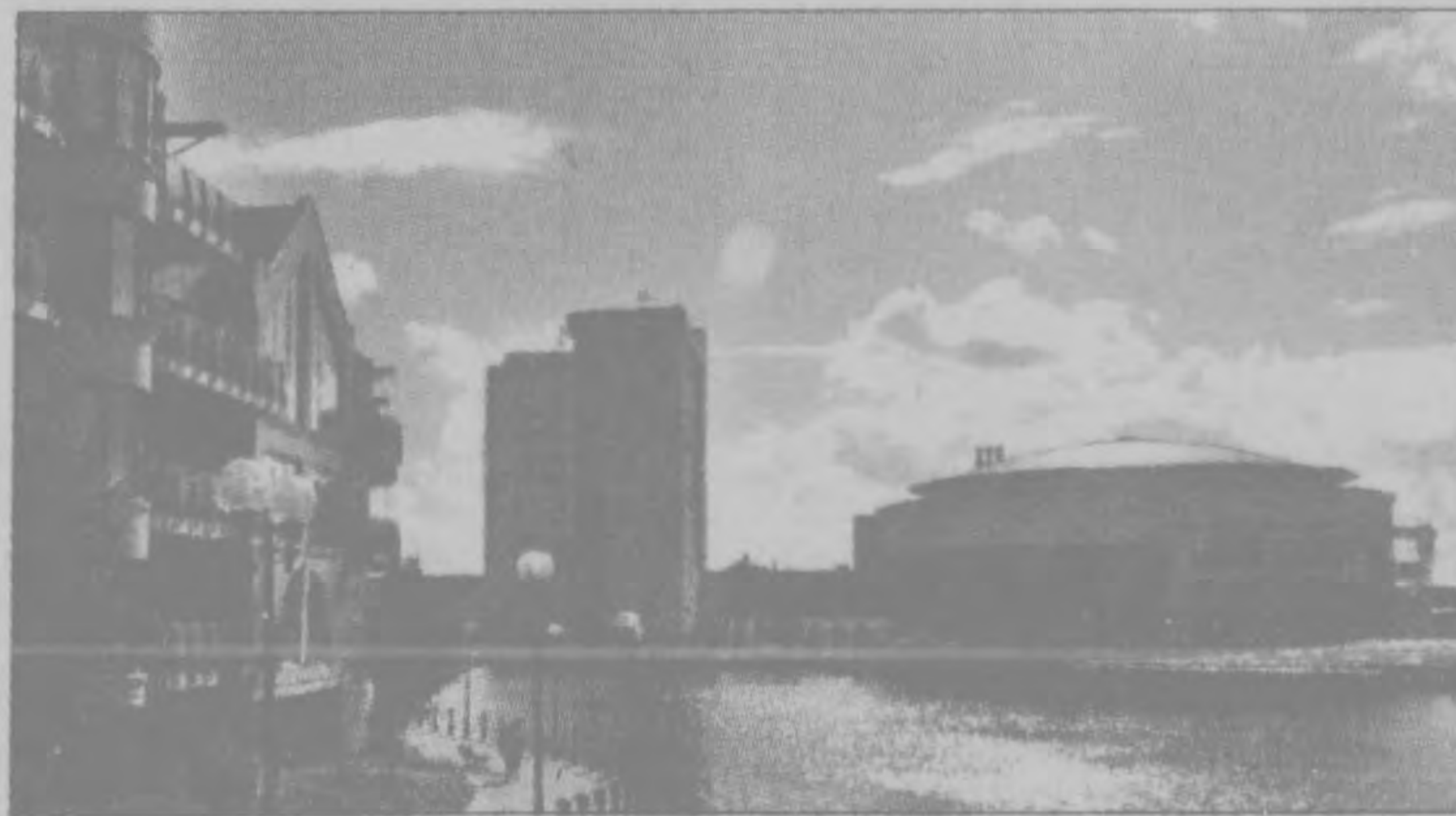
Along the River Lagan in Belfast, the Waterfront Hall is notable for a north side that is virtually all glass — an unthinkable concept a decade ago.
